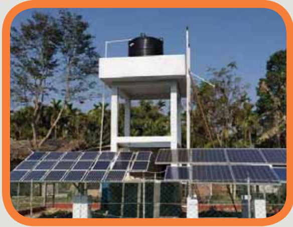
Solar Powered Drinking Water Plant (Project Rupkathar Gaon)
