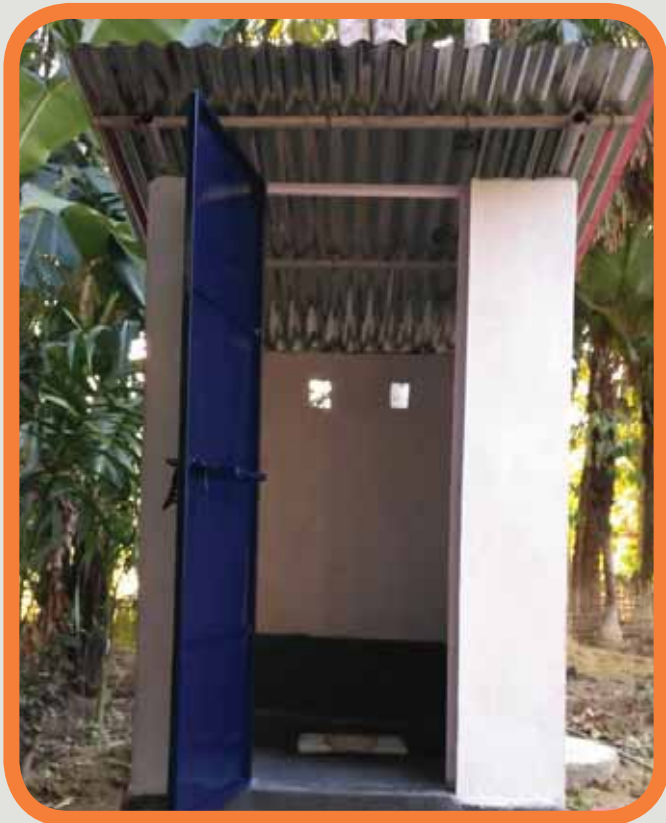
Toilet (Project Rupkathar Gaon)
